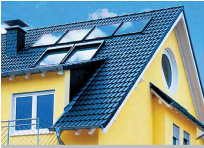
Solar hot water systems can supply most of a home's hot water without the use of fossil fuels. Israel is a world leader in solar water heating. (Credit: VELUX/ESTIF).
