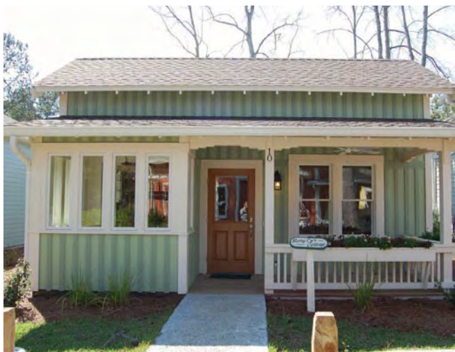
The Betty Lou Cottage, built by Coastal Habitats Construction and Development. This project utilized Earthcraft House green building guidelines with OneWorld Sustainable acting as the third party verifier and Energy Efficiency Consultant.
