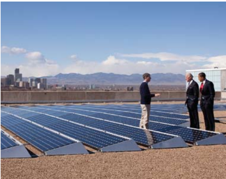
President Obama and Vice President Biden inspect solar panels on the roof of the Denver Museum of Nature & Science prior to the signing of the American Recovery and Reinvestment Act, which will provide a big boost to renewable energy projects.
