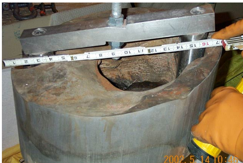
In 2002, corrosion of the vessel head at the Davis-Besse nuclear power plant in Ohio could have led to the loss of coolant from the reactor core and a meltdown. The incident is considered to be the most serious in the United States since Three Mile Island. (Photo: Nuclear Regulatory Commission)
