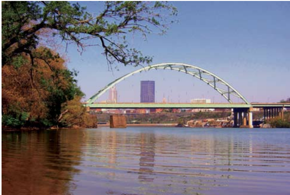
Ramps on the Birmingham Bridge fell about 8 inches after a problem with a key support mechanism, forcing an extended closure. Photo by Dave Gingrich.
