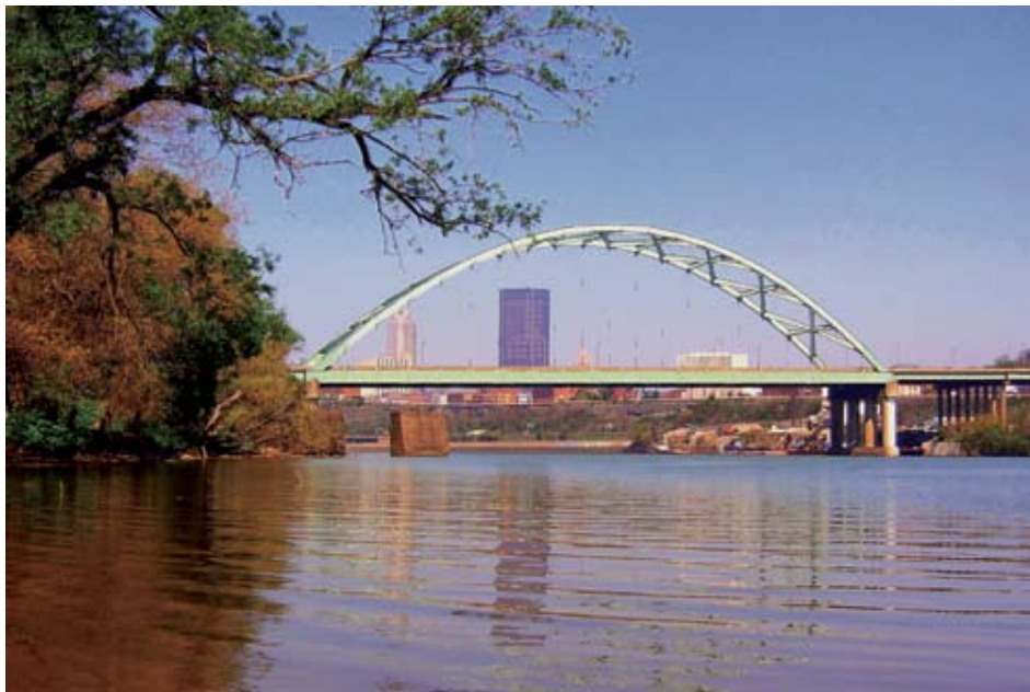
Ramps on the Birmingham Bridge fell about 8 inches after a problem with a key support mechanism, forcing an extended closure. Photo by Dave Gingrich.
