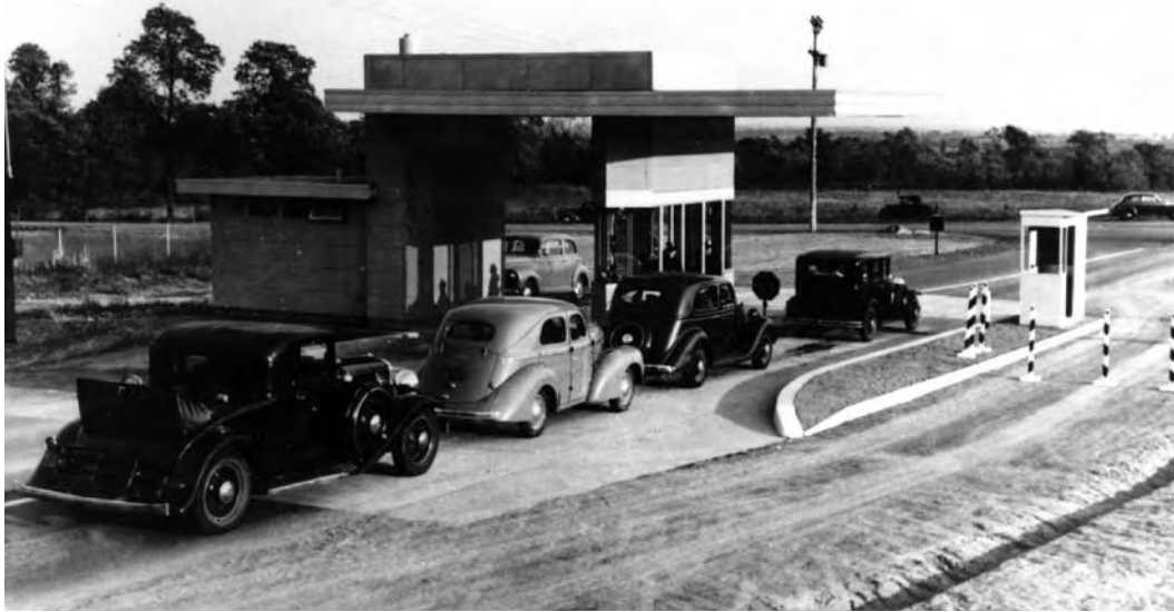
Drivers enter the Pennsylvania Turnpike, America's first superhighway, at its opening in 1940. Credit: Pennsylvania Turnpike Commission
