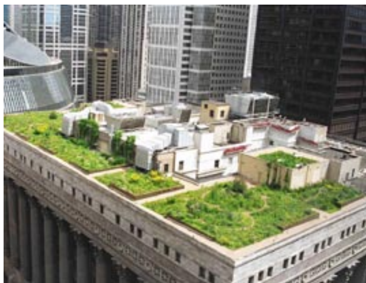
Chicago's City Hall was retrofitted with a green roof in 2000.
