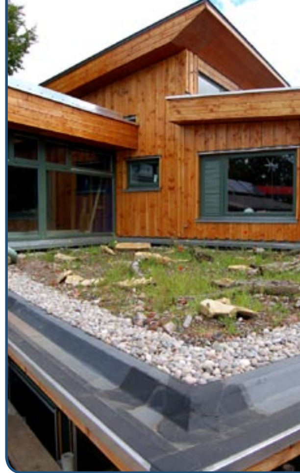
Green roofing is one of many ways to boost the energy efficiency of homes and office buildings.
