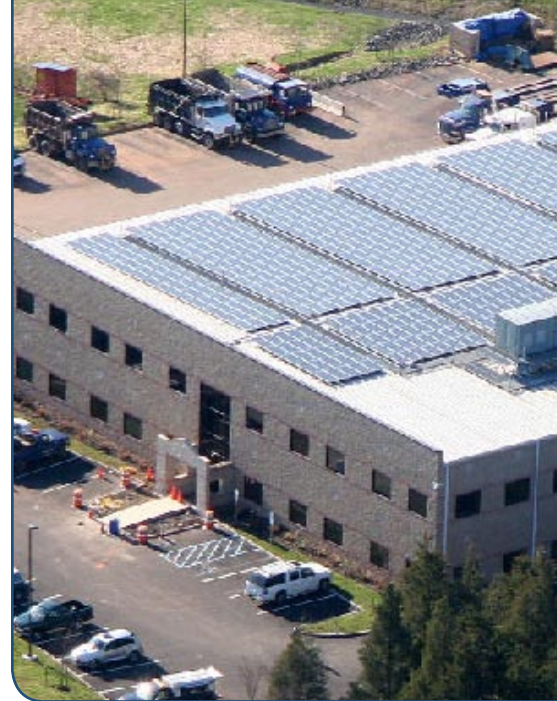
The Ferreira Construction building in New Jersey is the first zero electricity commercial building.
