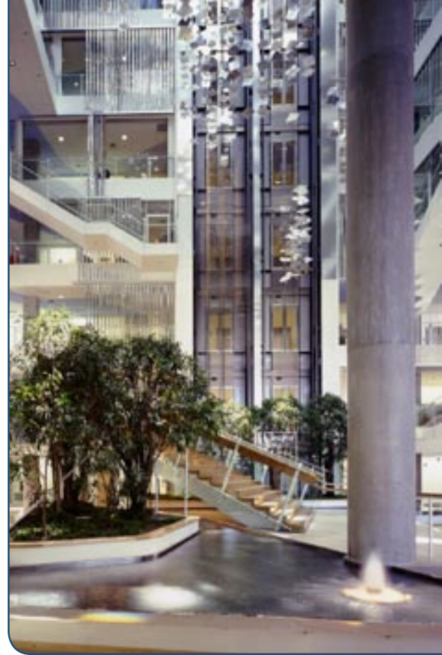
Genzyme, a biotechnology company, designed its corporate headquarters in Cambridge, Mass., to be extremely energy-efficient, with electricity costs about 42 percent less than a comparable building. Use of daylight allows 75 percent of employees to work with natural light alone. 12
