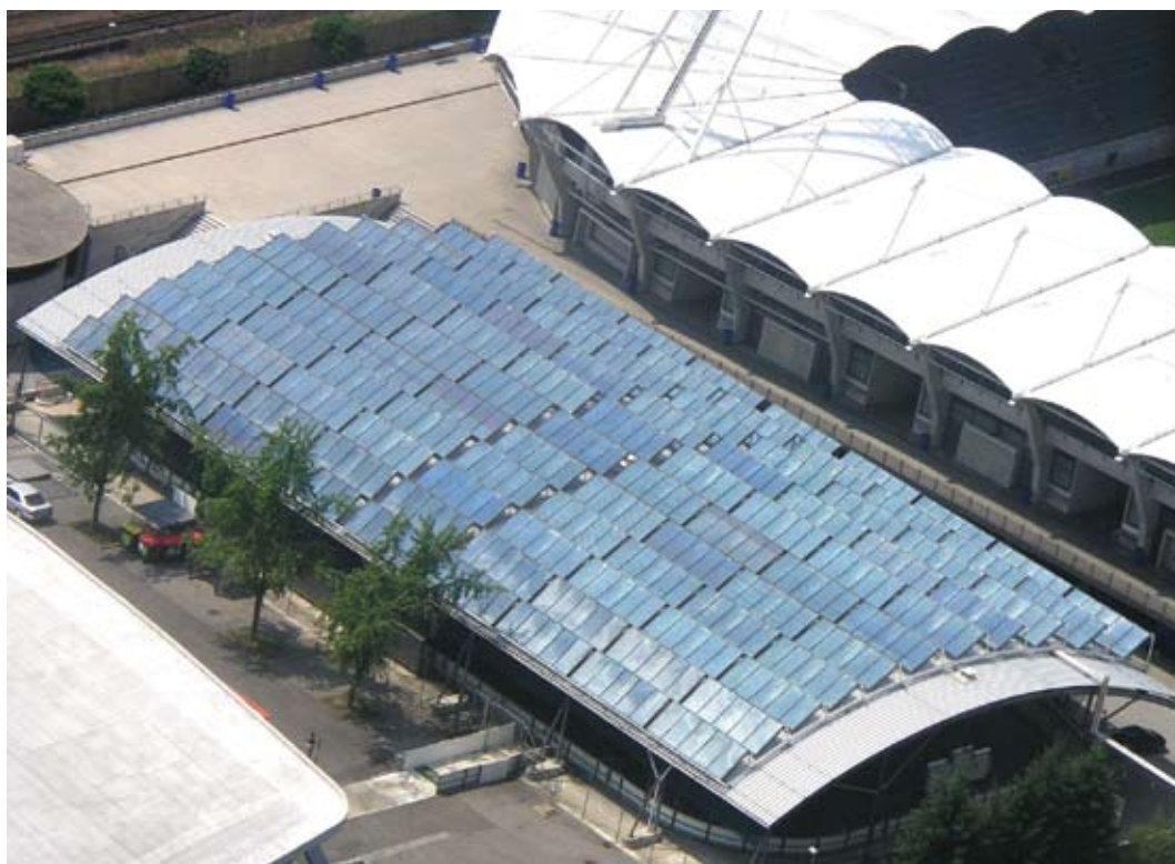
This solar thermal array, installed at Arnold Schwarzenegger Stadium in Graz, Austria, provides heat for the town's district heat system. Credit: SOLID/ESTIF
