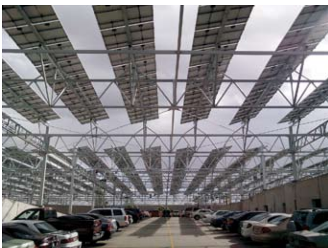
Solar garages, such as this one at Arizona State University, shade vehicles while providing power to the grid, and could someday be used to charge plug-in vehicles. Credit: Kevin Dooley, reprinted under Creative Commons license.
