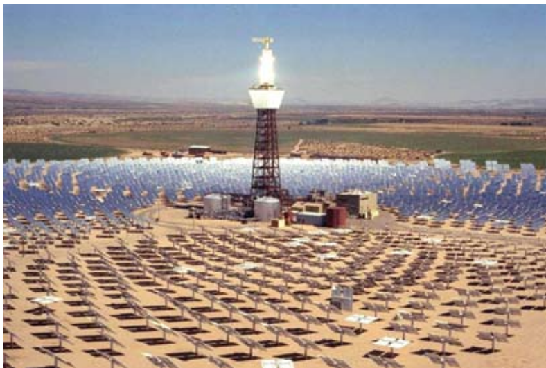
Solar “power towers” such as this one in California use arrays of mirrors to focus sunlight on a central receiver, and can incorporate thermal storage, which enables the plant to deliver electricity even at night. Credit: Sandia National Laboratory
