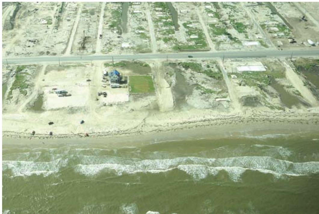
A lone house stands on a section of Texas' Bolivar Peninsula that was inundated by the storm surge from 2008's Hurricane Ike. Credit: Adam T. Baker
