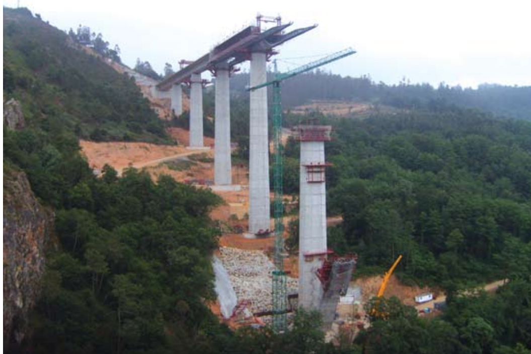
Construction of high-speed rail lines in other countries has created thousands of jobs. Here, construction is underway on a bridge as part of Spain's efforts to extend its high-speed rail network. Credit: Xosema, used under Creative Commons license
