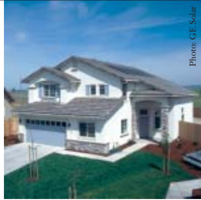
A home fitted with rooftop solar panels.
