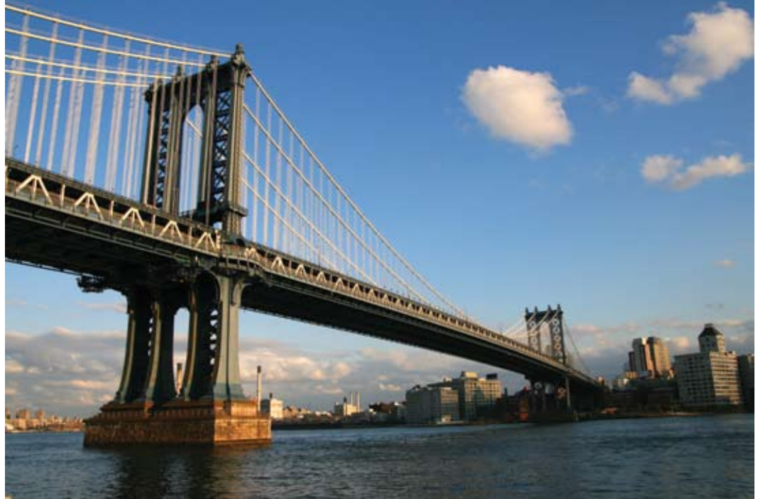
The Manhattan Bridge in New York City. Photo by Tim Schnurpfeil
