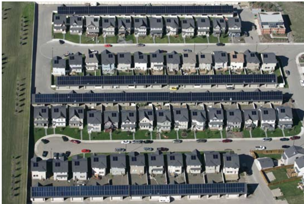
Solar water heating can work in any climate. In Alberta, Canada, the Drake Landing housing development is equipped with a solar district heat system that serves the majority of the complex's heat and hot water needs. Credit: Natural Resources Canada
