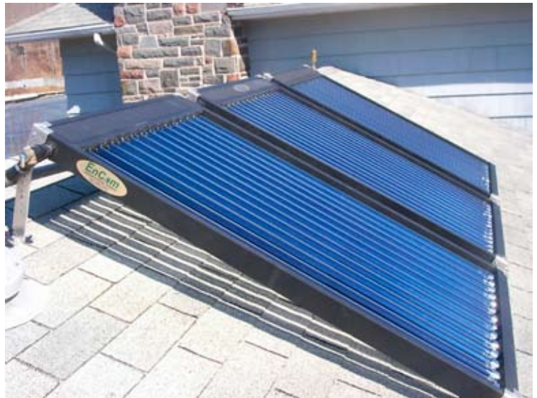
Solar water heating systems can reduce electricity or fossil fuel use for water heating by about two-thirds.
