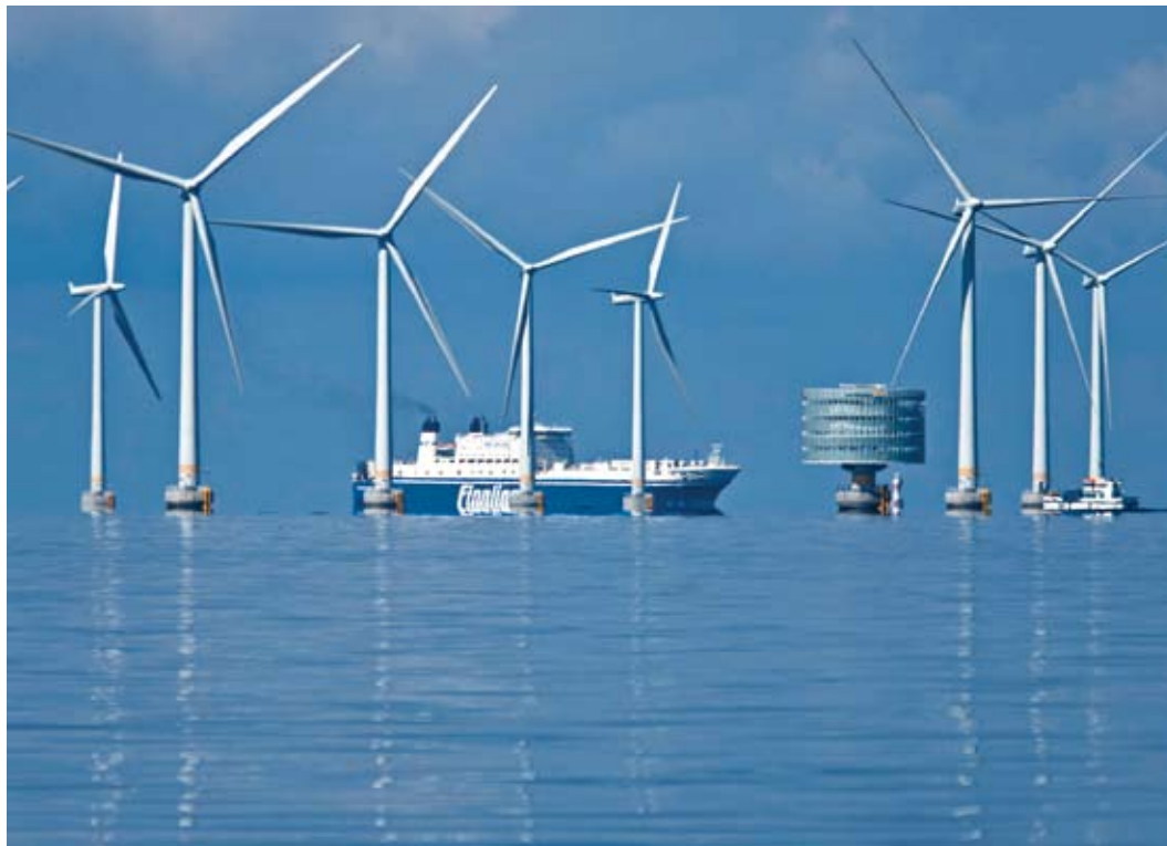
Offshore electrical substations, such as the cylindrical structure above, aggregate the electricity generated by the individual wind turbines, where it can be delivered via submarine cables to the shore. Credit: Siemens
