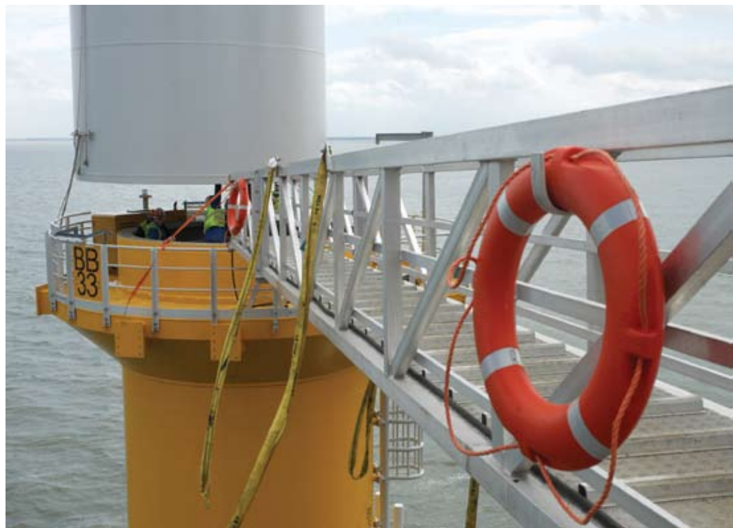
Foundations are massive steel structures, weighing hundreds of tons, that root offshore wind turbines to the seafloor. Foundations are typically fabricated locally, given the cost and difficulty of transporting them long distances. Here, an offshore wind turbine in the United Kingdom is affixed to its foundation. Credit: Siemens
