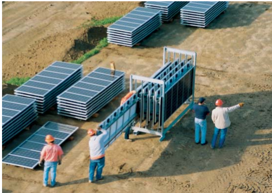
Construction workers prepare to install solar panels.
