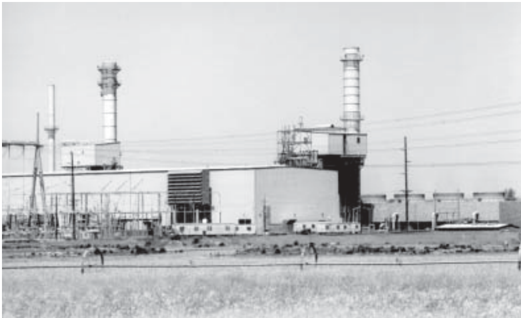
A natural gas power plant.
