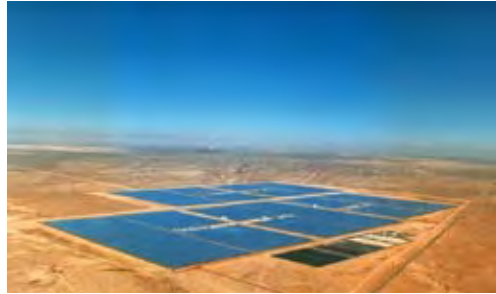
An aerial view of the parabolic trough arrays at Kramer Junction, California. The five facilities have a combined production capacity of 150 MW. (Credit: Gregory Kolb, Sandia National Laboratories)
