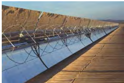
A row of parabolic trough solar collectors in a 150 MW parabolic trough solar thermal array in California. (Credit: Gregory Kolb, Sandia National Laboratories)
