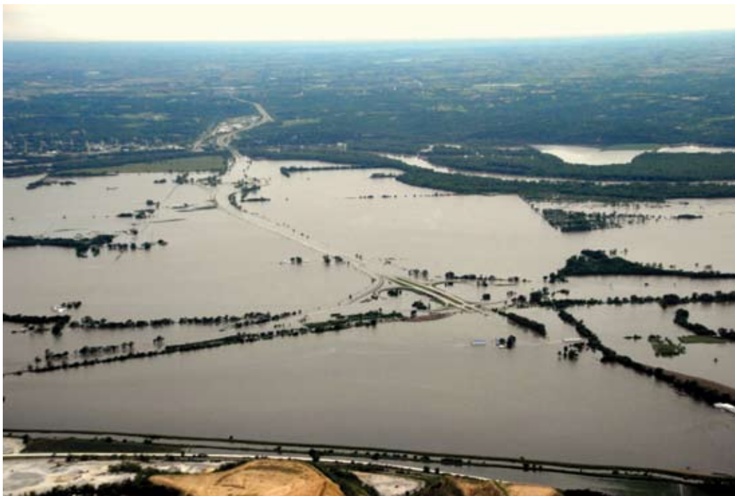
In June 2011, massive flooding along the Missouri River—fueled by snowmelt and runoff from an unusually large number of extreme storms in the watershed that spring—inflicted as much as $1 billion worth of damage to the region’s flood control system and inundated several miles of Interstate 680, including the intersection of I-29 and I-680 by Mormon Bridge in Council Bluffs, Iowa (pictured here). Credit: U.S. Army Corps of Engineers
