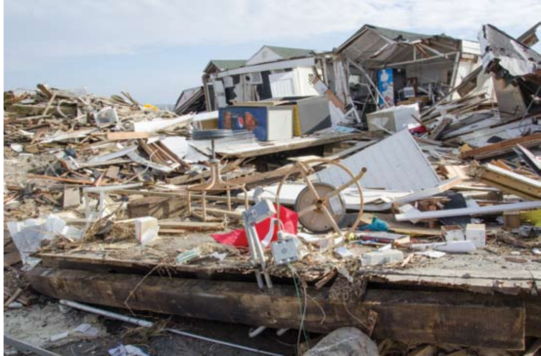
Hurricane Sandy caused extensive damage in the Northeast, including at this location in Deal, New Jersey. Credit: FEMA
