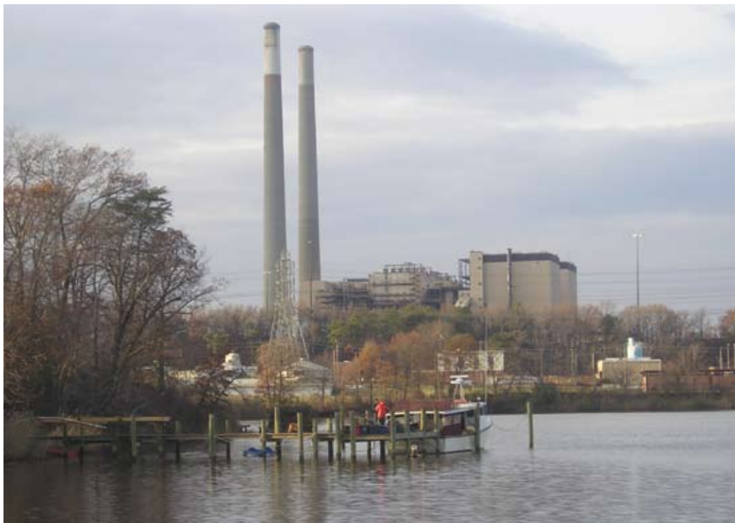
The Brandon Shores coal-fired power plant in Maryland is one of the facilities regulated by RGGI.
