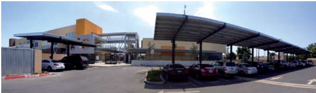
This 116 kW solar carport system was installed at the South Region Elementary School as part of the Los Angeles Unified School District's commitment to clean energy. Credit: Los Angeles Unified School District
