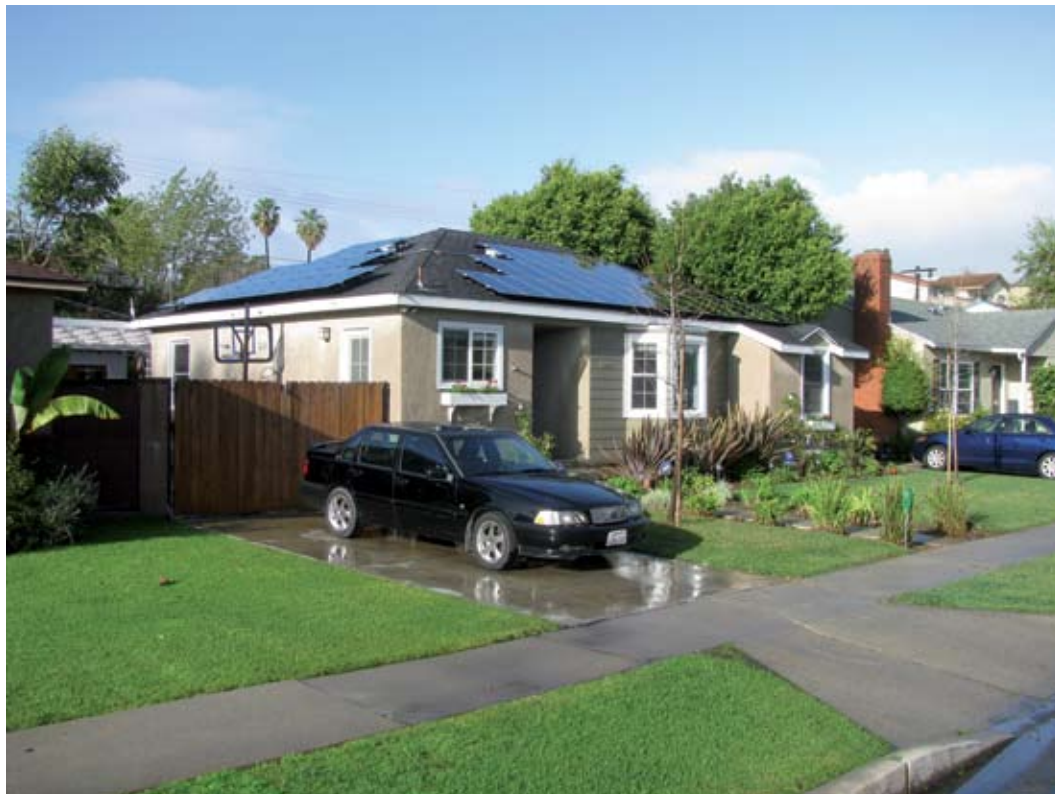
This residence in the Mar Vista area of Los Angeles benefits from a 3.9 kW thin-film solar array. Credit: John Ayers
