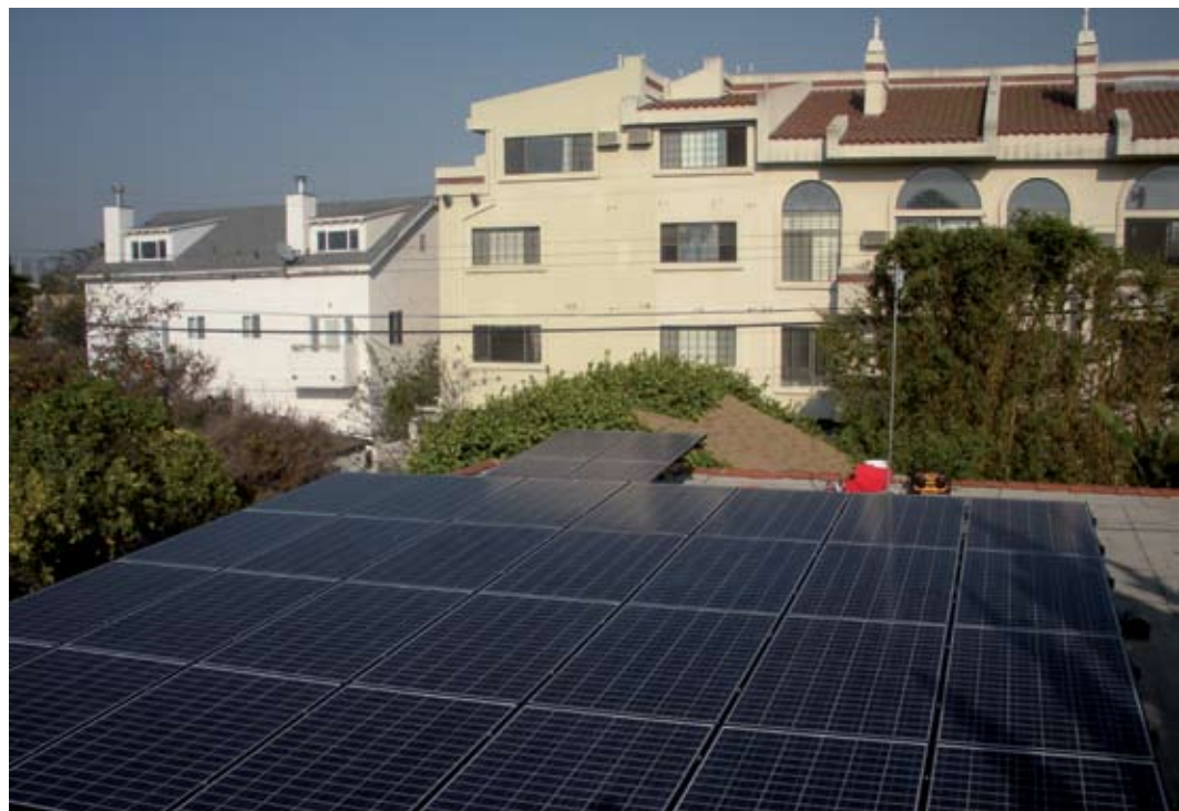
A 6.5 kW solar array offsets 90 percent of the energy needs of this building in the Mar Vista area of Los Angeles. Credit: Sarah Auerswald
