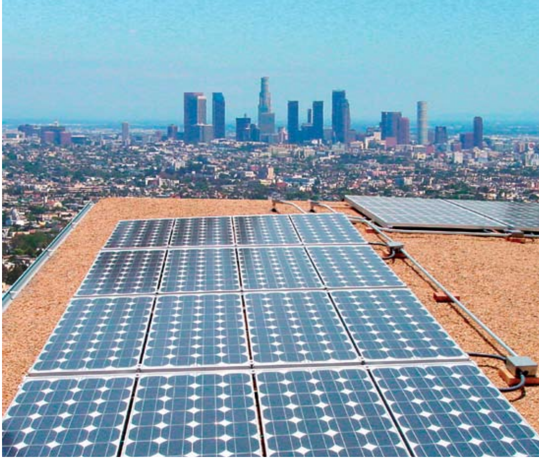
This residential solar array overlooks the downtown Los Angeles skyline. Credit: Graham Owen, Ameco Solar
