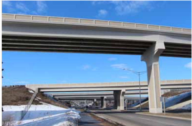
Soaring ramps mark the newly expanded Interstate 39/U.S. Highway 51/State Highway 29 in Wausau.
