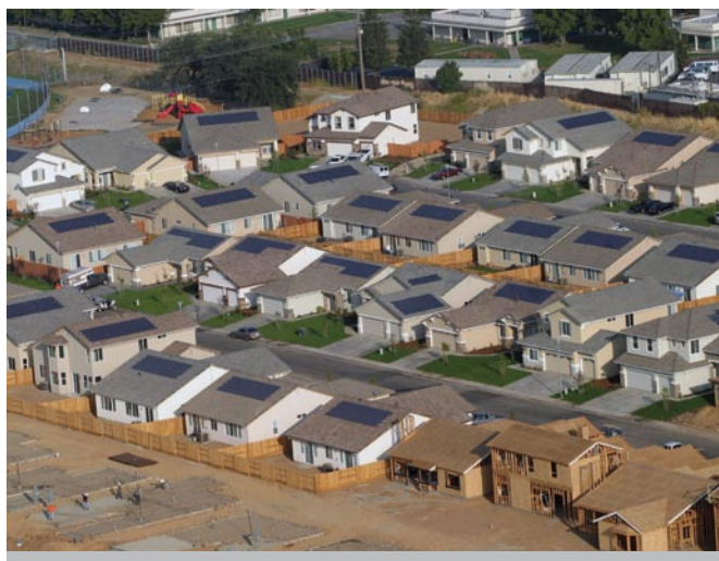
Zero energy homes, like those under construction in this Sacramento subdivision, couple energy-efficient design with small-scale renewable energy generation to dramatically reduce consumption of fossil fuels. (Credit: Sacramento Municipal Utility District)
