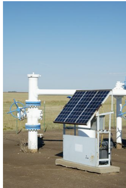
The oil and gas industry is the largest user of PV. Here, solar panels power the monitoring equipment on a pipeline in the Texas Panhandle.
