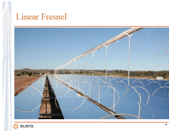
A linear Fresnel reflector solar thermal power plant. (Credit: Ausra)
