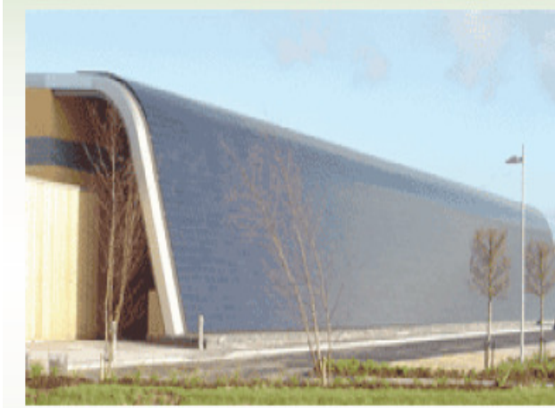
Thin-film PV “skins” can be used to turn the exterior surfaces of buildings into power plants. Credit: HelioVolt Corporation
