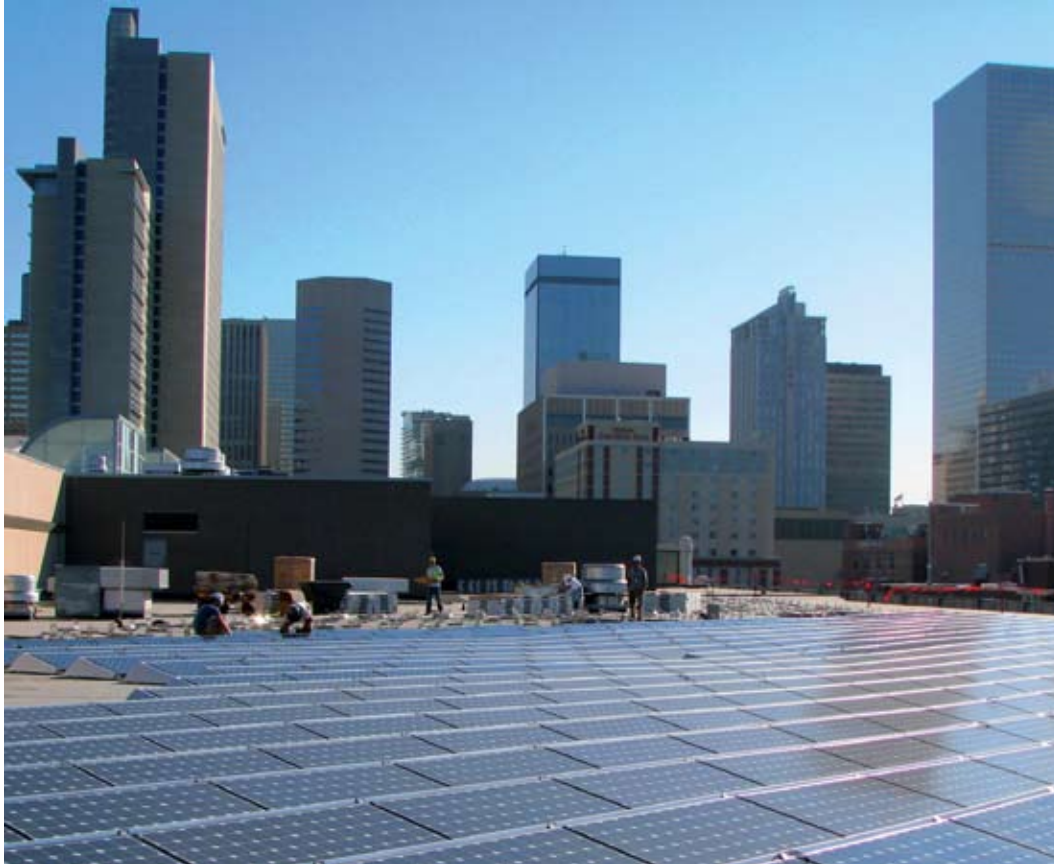
Namaste Solar Electric installs a 300 kw PV rooftop installation on top of the Colorado Convention Center in Denver in March 2012.
