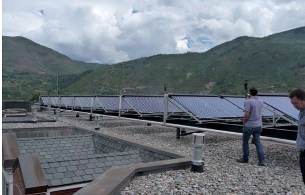
Rooftop solar water-heating system above the Grand Hyatt resort in Aspen.
