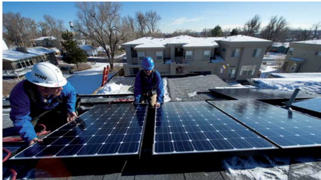
Two installers with Lighthouse Solar put microcrystalline PV modules on top of a townhome in Golden in December 2011.
