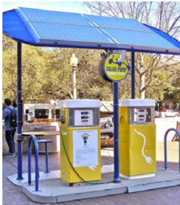
This electric car charging station is powered by solar panels installed on the roof.
