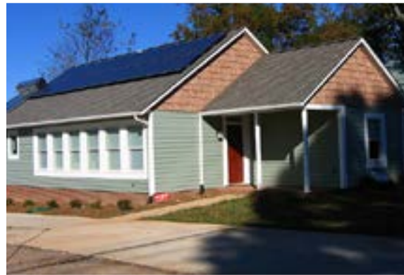
Energy efficient home with solar panels installed on roof.
