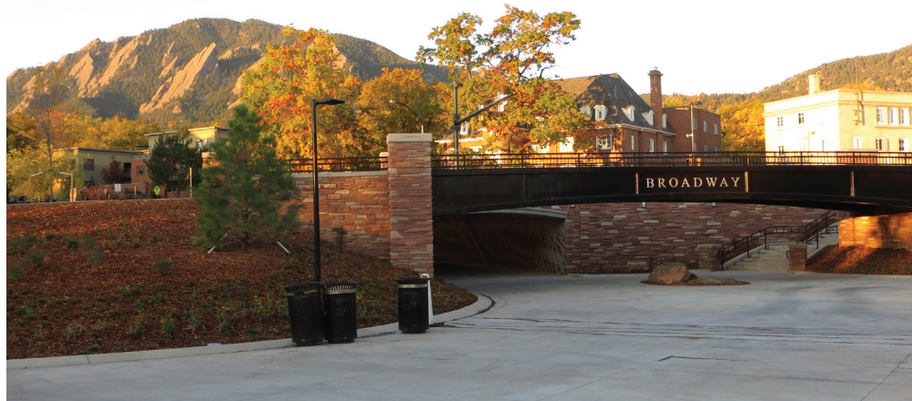
Pedestrian and bicycle underpass at Broadway bordering the CU-Boulder campus.
