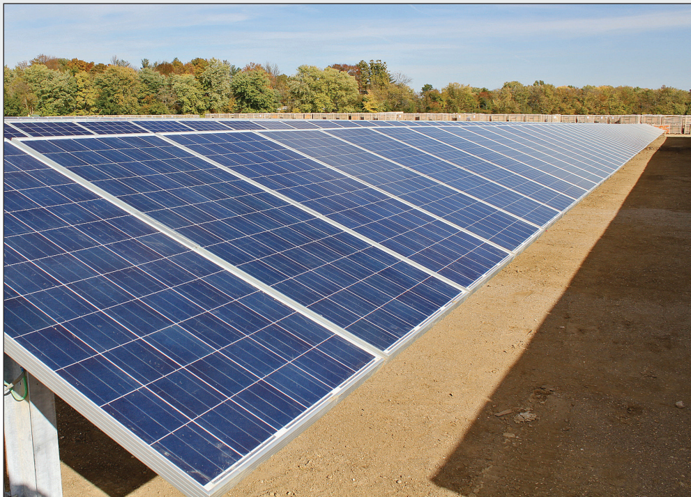
The "Indy I" Solar Array depicted is one of three utility-scale solar projects owned by Dominion Energy Resources—these projects represent a combined 28.6 MW of solar power in Indianapolis.
