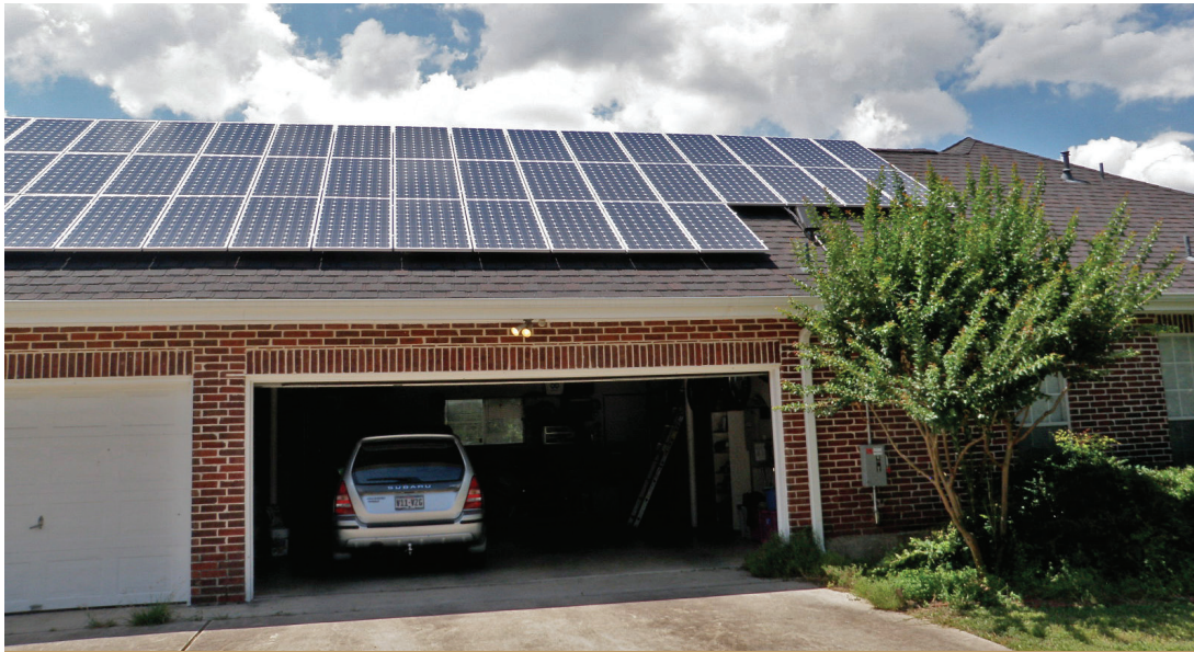
A solar energy system installed on the roof of a house in San Antonio with the help of CPS Energy.
