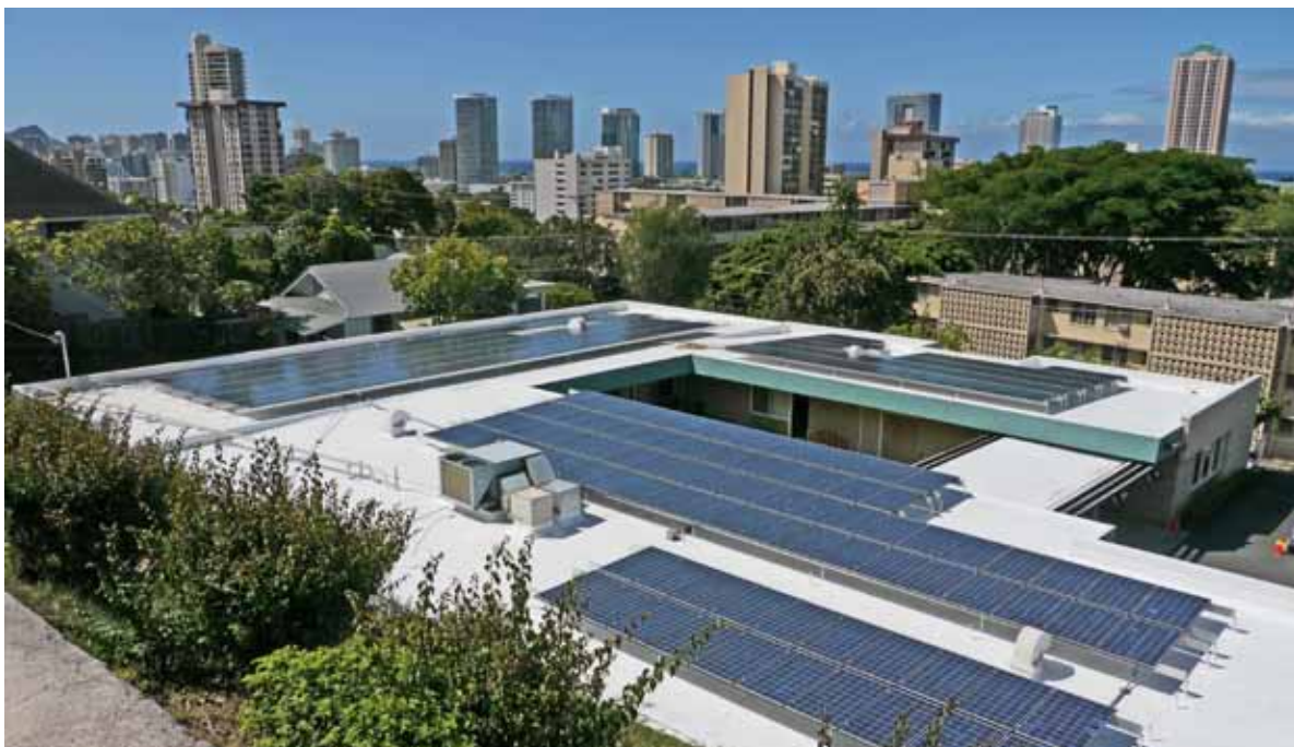
Solar panels on the roof of the non-profit Easter Seals Society building with downtown Honolulu in the background.
