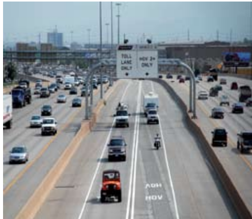
Express lanes on I-25 in Denver. The Colorado Department of Transportation wants to add express lanes to C-470 south of the city.
