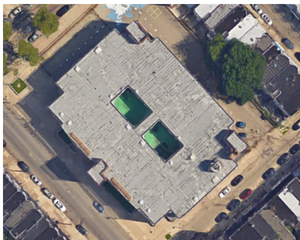
Figure 4. Thomas Morton Elementary School Has the Median Rooftop Solar Panel Space Among Philadelphia Schools
