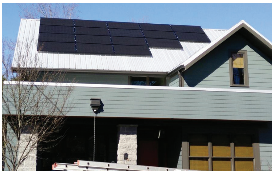
Solar panels on a home in Athens, GA.
