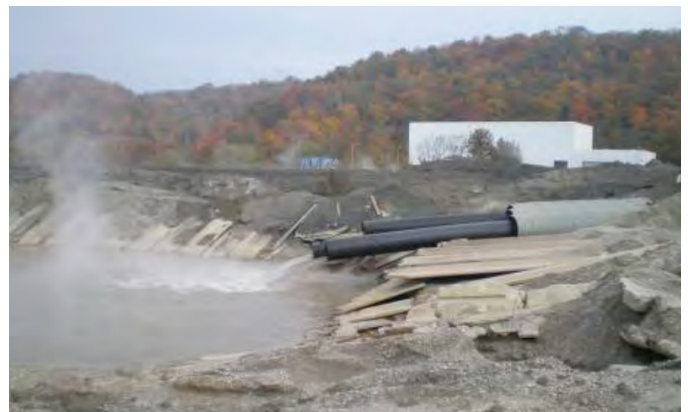
Sluice lines entering “Pond 5” at the J.M. Stuart Station, located in an Ohio River flood zone. Pond 5 was found by an EPA assessment to be in “Poor” condition, and to pose a “Significant” hazard to the surrounding area. Image: EPA
