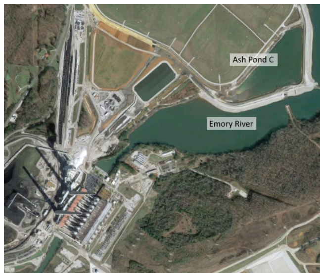
At the Kingston Fossil Plant, Ash Pond C contained decades worth of toxic coal ash waste. When the coal ash pond's dike failed, more than 1 billion gallons of coal ash waste flowed into the nearby Emory and Clinch rivers. 12 Image: U.S. EPA
