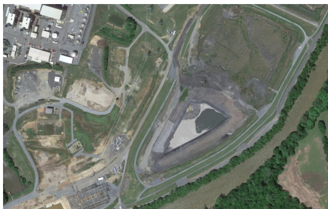
Overhead view of ash ponds at the Dan River Steam Station. Imagery ©2018 Google
