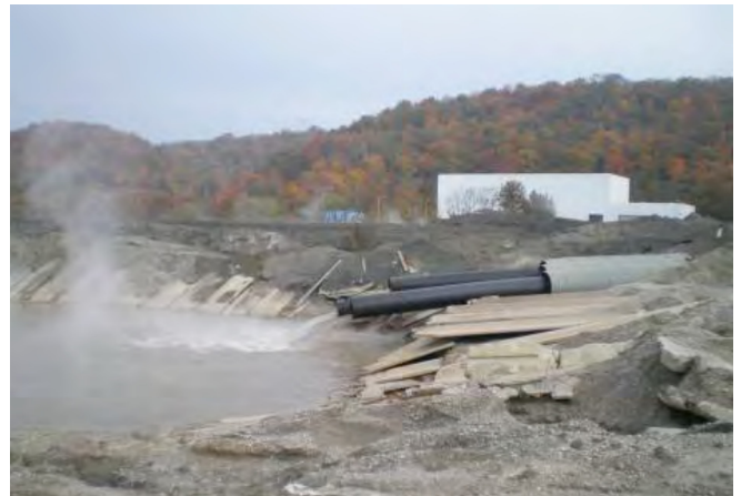
Sluice lines entering "Pond 5" at the J.M. Stuart Station, located in an Ohio River flood zone. Pond 5 was found by an EPA assessment to be in "poor" condition, and to pose a "significant" hazard to the surrounding area. Image: U.S. Environmental Protection Agency
