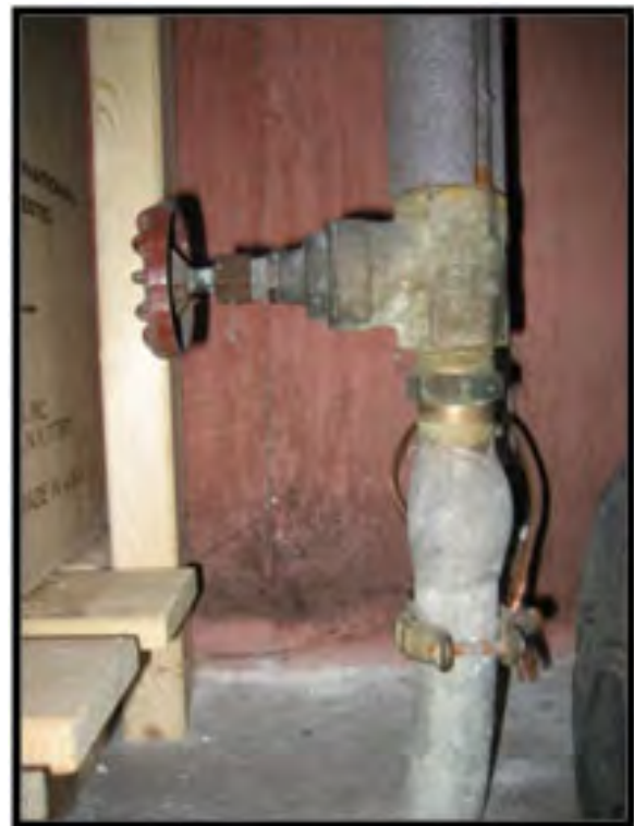
A Lead Service Line 58 Credit: EPA
