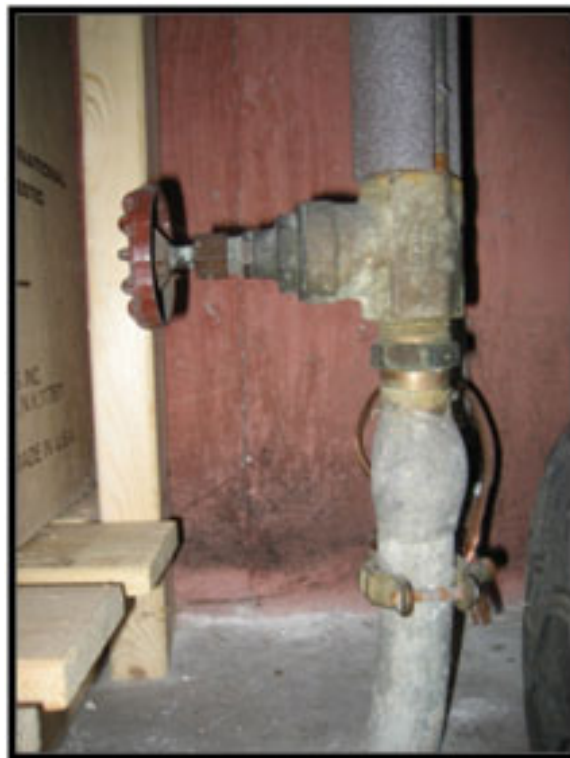
A Lead Service Line 58 Credit: EPA
