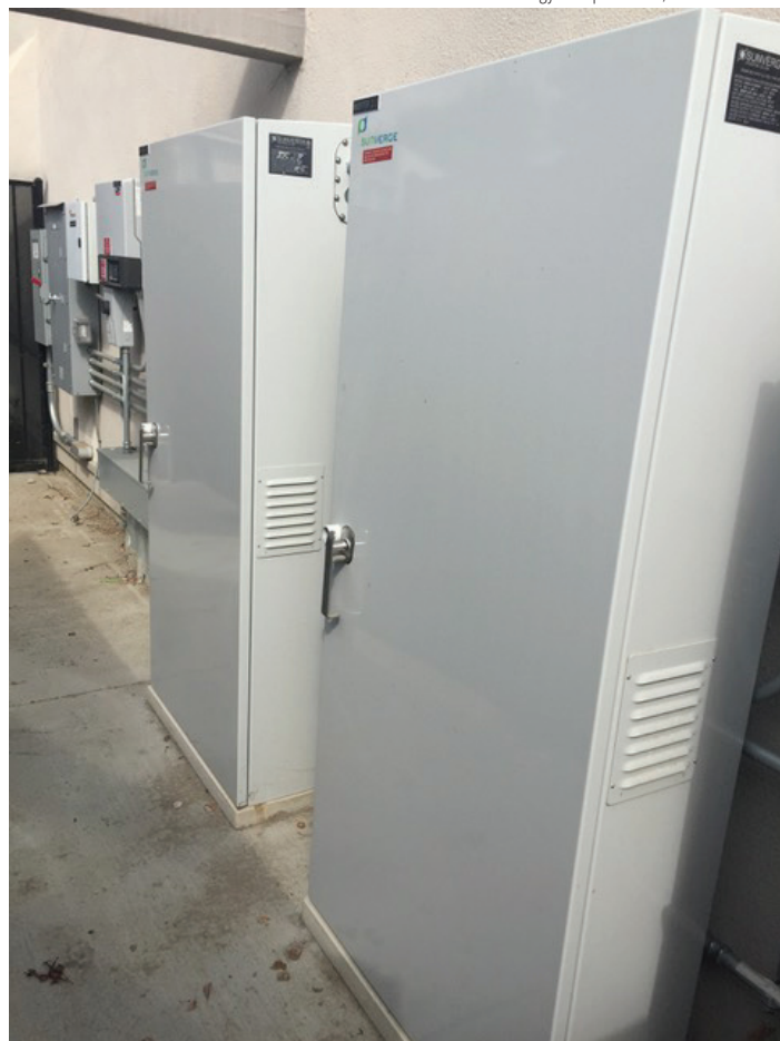
“Behind-the-meter” battery storage at an apartment complex in Los Angeles County, California.
