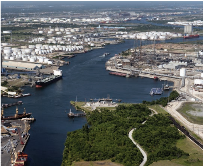
The Houston ship channel and petroleum facilities.
