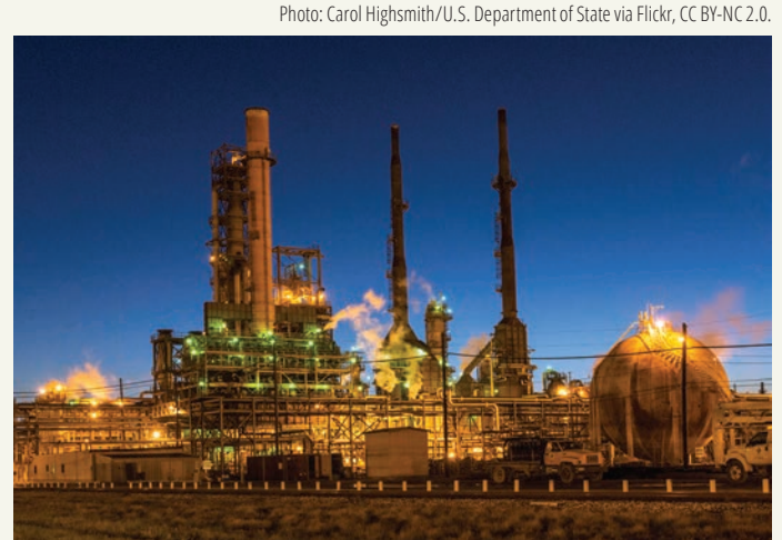
The Valero refinery in Port Arthur, Texas, at dusk.
