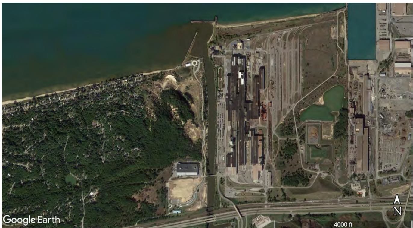
This U.S. Steel Corporation plant on the shore of Lake Michigan spilled hexavalent chromium, forcing the closure of adjacent beaches. Image: ©2018 DigitalGlobe, IndianaMap Framework Data, Landsat / Copernicus, U.S. Geological Survey, USDA Farm Service Agency
