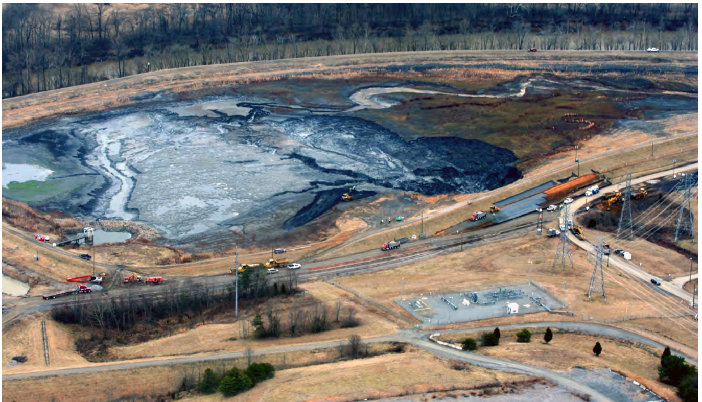
Coal ash spill into the Dan River in North Carolina, 2014. Image: Waterkeeper Alliance/Rick Dove on Flickr (CC BY-NC 2.0)
