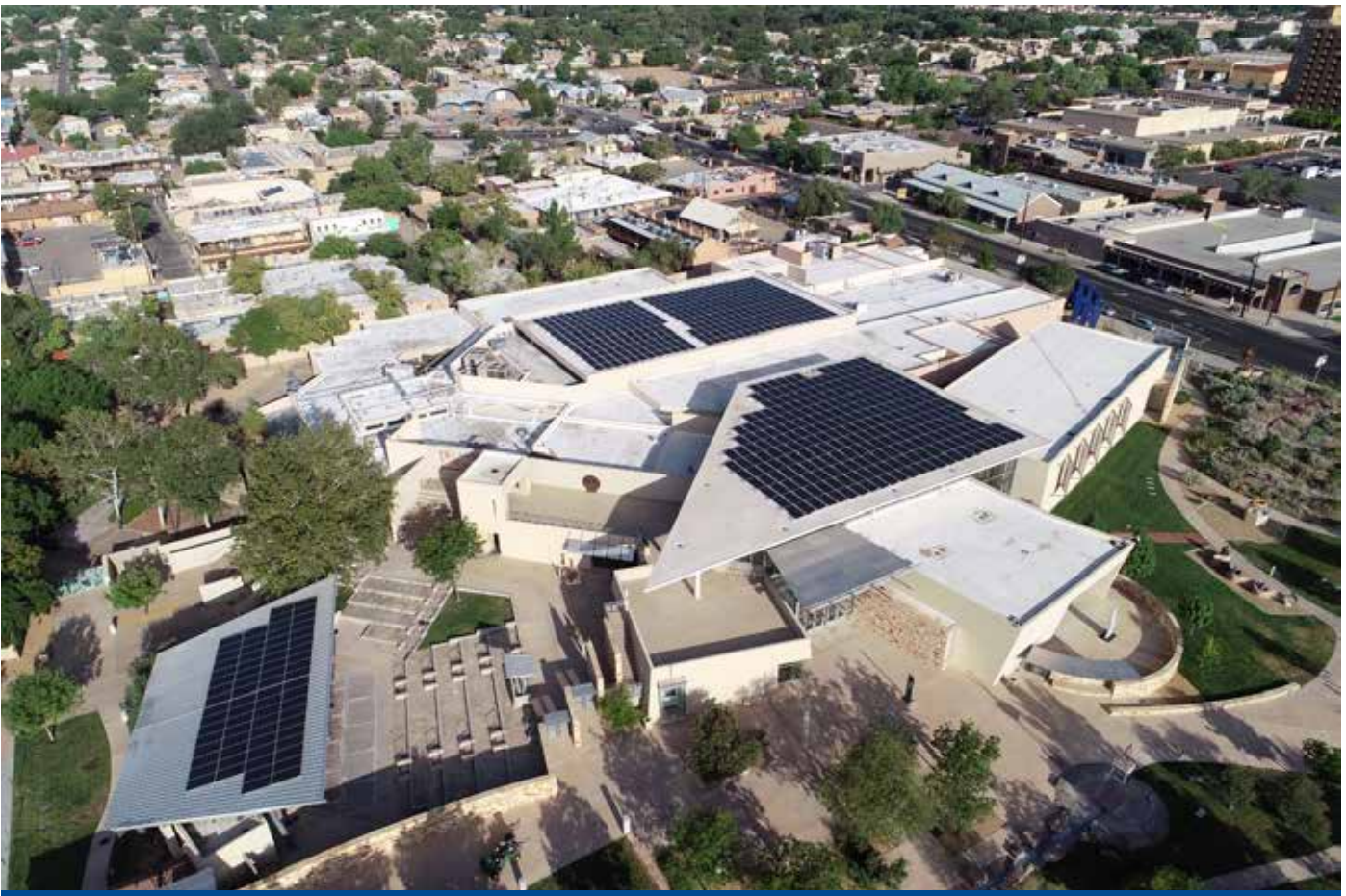
Rooftop solar panels on the Albuquerque Museum.
