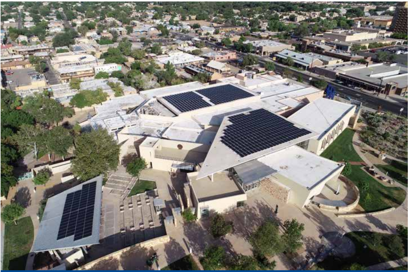
Rooftop solar panels on the Albuquerque Museum.
