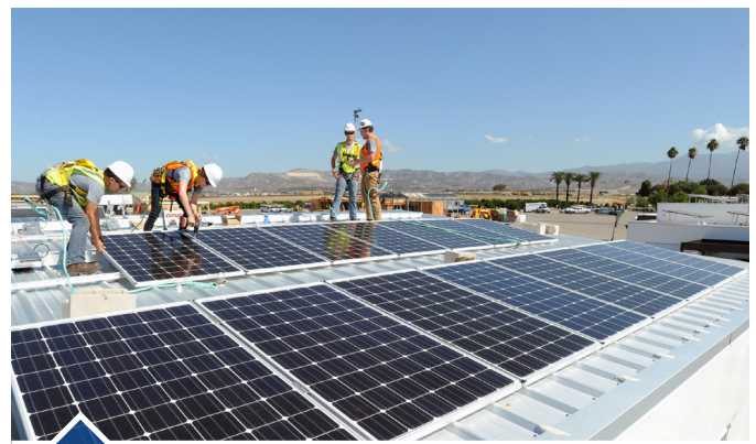
Solar panels being installed in California.
