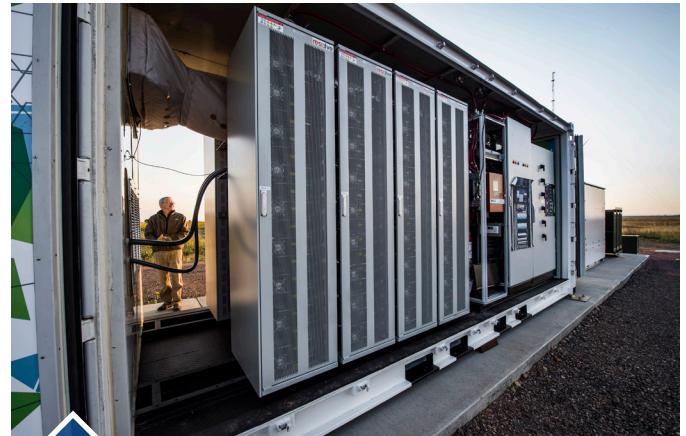
Battery storage can help to integrate more renewable energy into the grid.
