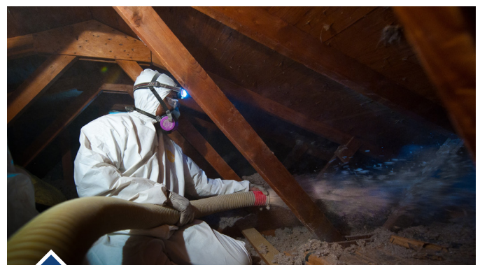
Home weatherization saves energy and money.
