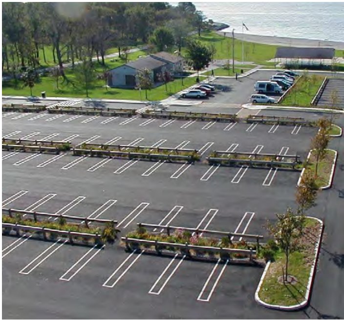
Green Stormwater Infrastructure in Town Beach Parking Lot, Bristol Rhode Island. Credit: Rhode Island Department of Environmental Management
