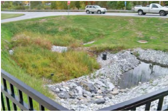
St. Albans Gravel Wetland after completion. Credit: Watershed Consulting
