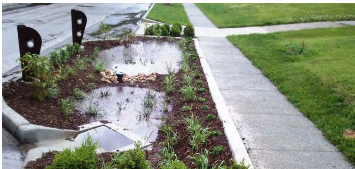
Vegetated stormwater retention basin, curb extension. Credit: Kansas City Water Services
