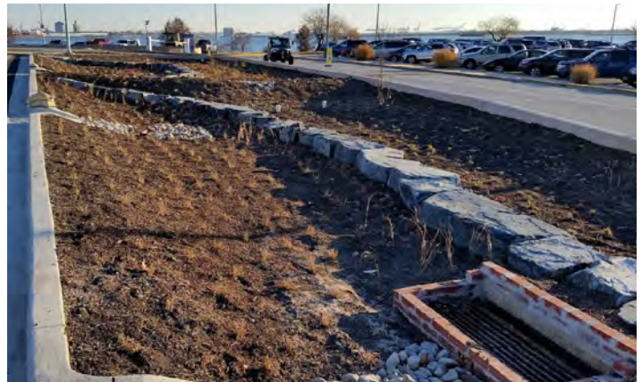
Vegetated stormwater basin in parking lot after planting. Credit: Blue Water Baltimore
