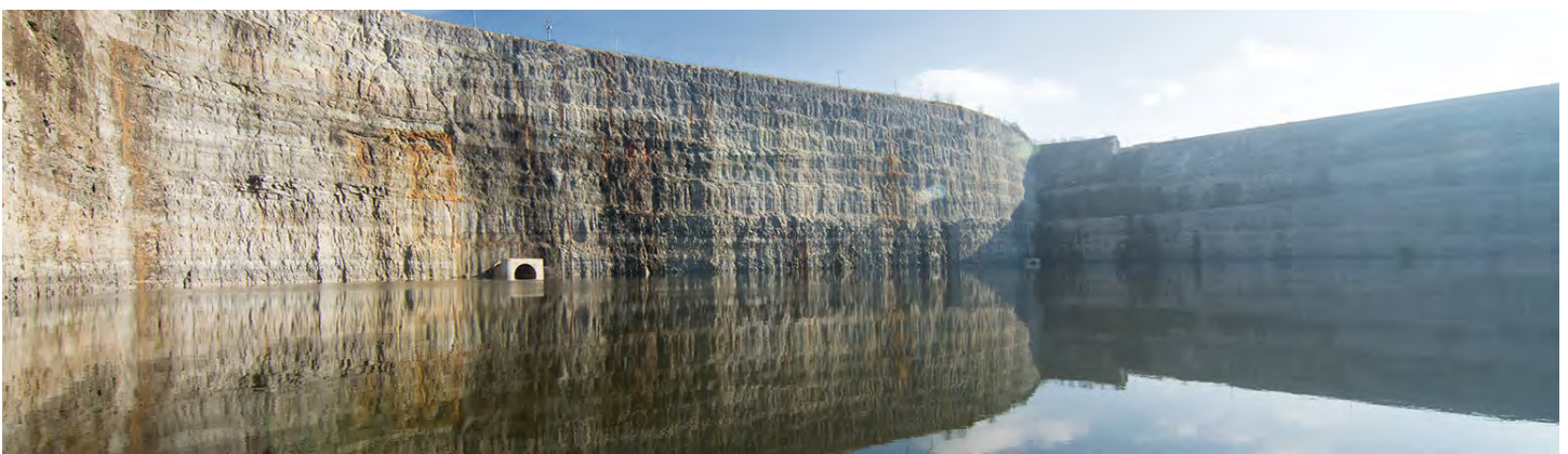
TARP Reservoir, Credit: MWRD
