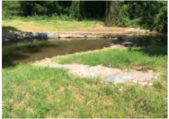
Mill Creek erosion control. Credit: EPA
