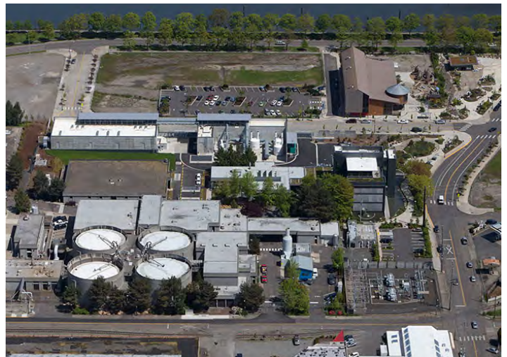
Budd Inlet wastewater treatment plant. Credit: LOTT Clean Water Alliance
