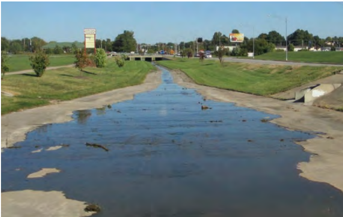
South Creek before restoration. Credit: City of Springfield and James River Basin Partnership
