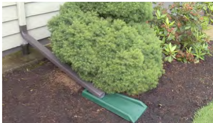
Downspout disconnection as part of the Cornerstone Projects. Credit: City of Portland
