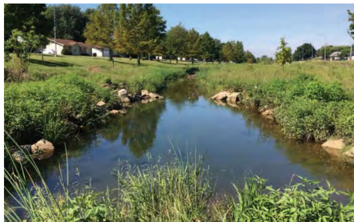
South Creek after restoration, with vegetated stormwater filtration systems at outfalls along creek. Credit: City of Springfield and James River Basin Partnership
