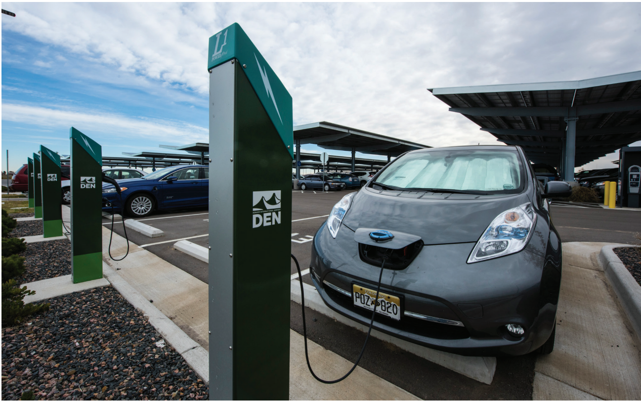
This electric vehicle charging station is powered by solar panels installed on a parking canopy. Because electric vehicles can be powered by clean energy sources including wind and solar power, they can enable a transition to a zero-carbon transportation future. Photo: Dennis Schroeder, National Renewable Energy Laboratory
