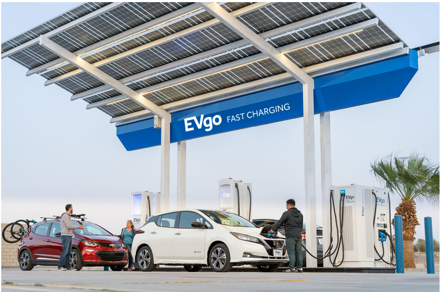
EV charging stations powered by solar panels can expand access to renewable energy for car charging. Credit: EVgo
