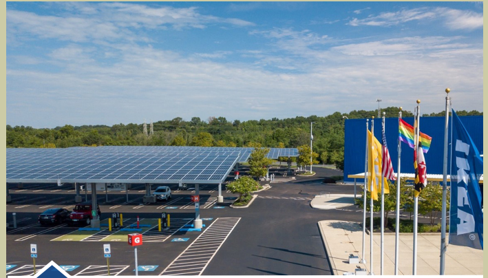
Solar parking canopy at IKEA in Baltimore, MD.
