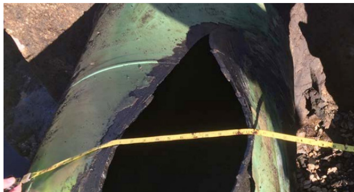
This Keystone Pipeline rupture in South Dakota led to the spill of approximately 5,000 barrels of oil.
