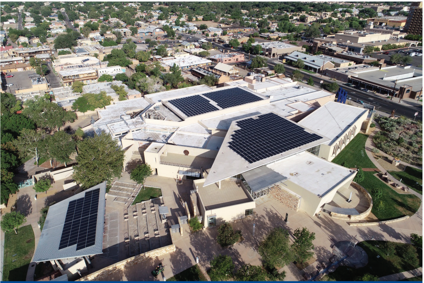
Rooftop solar panels on the Albuquerque Museum.
